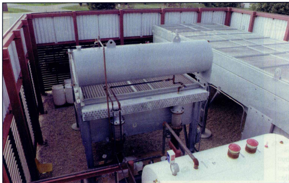
Adjacent to the cogeneration facility is a fenced area containing horizontal cooling units from Amercool that provide cooling for engine jacket water and intercoolers.
